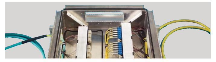
**Wiremold**<sup>®</sup> RFE Series Raised Floor Zone Cabling Enclosures create an intermediate or remote consolidation point that may be tested and secured prior to adding drops for voice and data outlets.
