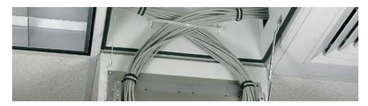
**Wiremold®** CZE Series Ceiling Zone Cabling Enclosures create an intermediate or remote consolidation point that may be tested and secured prior to adding drops for voice and data outlets.
