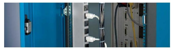
Power Commander<sup>®</sup> Series High Amperage Units (PDUs) have multiple circuits to provide increased capacity for today's high density server racks. Embedded or remote ammeters are available to monitor current draw.
