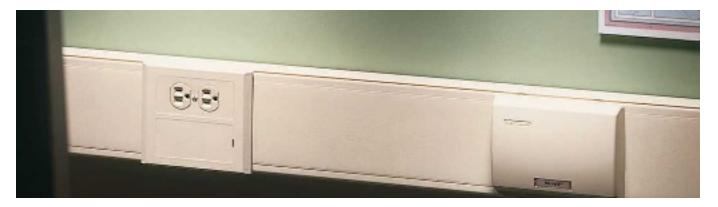
Large capacity, multiple channel raceway. Lightweight and easy-to-cut. Ideal for power or communication installations that require multiple services.
