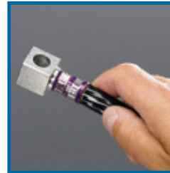
1. Crimp Multi-Tap connectors onto de-energized cables.
