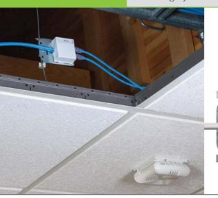
An In-Ceiling System provides a fixed location for terminating a data connector, creating a more reliable and consistent connection than a direct connect plug. This fixed connection also reduces the possibility of damage during construction.
